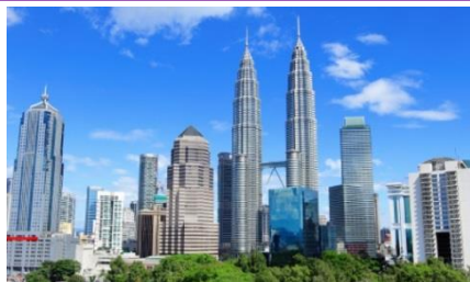
Petronas Twin Towers
